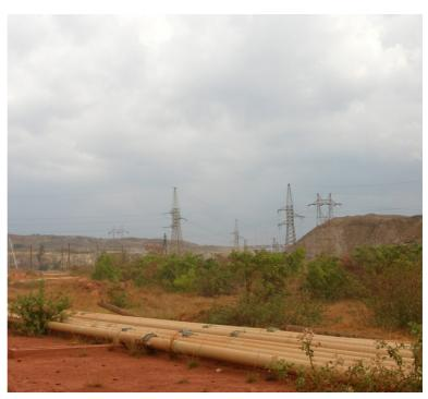
IN THE FOREGROUND, THE WHITE PIPES TRANSPORTING THE ORE FROM THE KAMOTO CONCENTRATOR TO THE LUILU HYDROMETALLURGICAL PLANT. IN THE BACK, THE DARKER PIPES CARRYING WATER TO LUILU AND WHICH HAVE BEEN PUNCTURED AND STOLEN.
